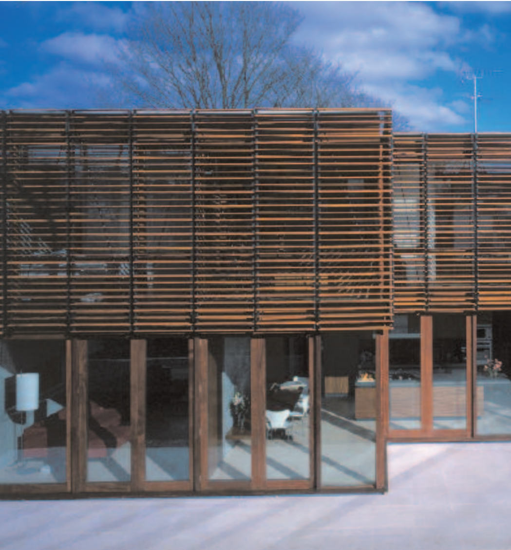
House in Aberdeen Lane, London N1, Azman Owens Architects. © Keith Collie
