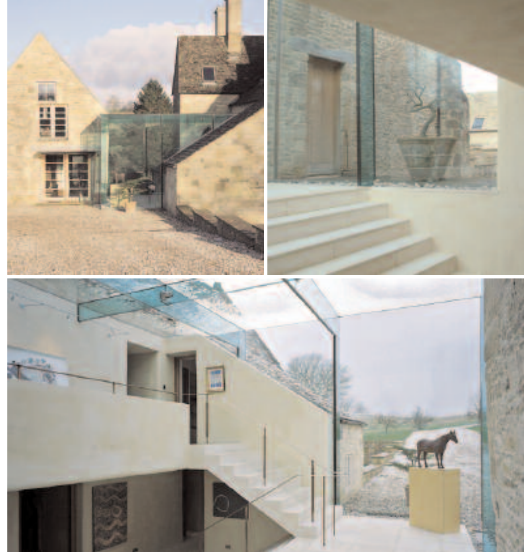
Private House, Gloucester, Jamieson Associates Architects. © Nick Meers
